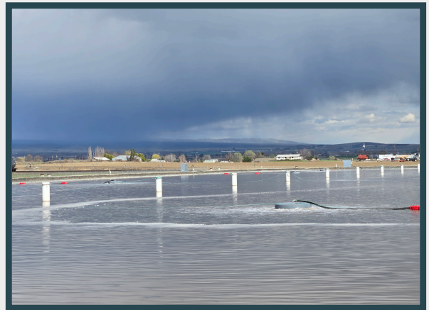
New Aerators Installed in Lagoon 2/3
